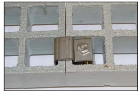
Installed G clamp
